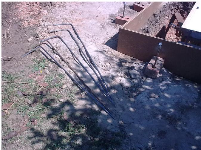
Extra steel starter bars were also ready to be placed into the wet concrete to further tie in and reinforce the whole tower base.
