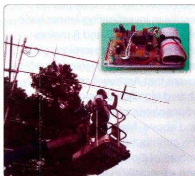
This month's cover The 7 MHz traps being installed on the HARG HF beam. See VK6 News on page 41. Inset: A view inside the low distortion two tone audio oscillator by VK5JST. See page 14. Main photo by Bill Rose VK6WJ, inset by Jim Tregellas VK5JST.
